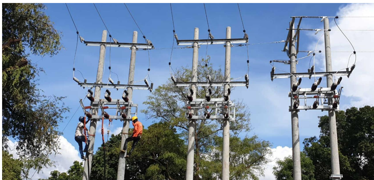
Figure 3.3: Technicians working on Juba’s Distribution Network in 2019
